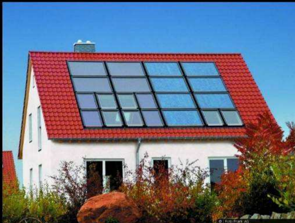
Left: combined solar thermal system for DHW and room heating support Right: PV system, combined with skylights
